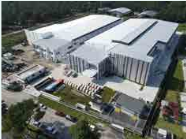
Design & Build Detached Factory for Shimano Malaysia.
