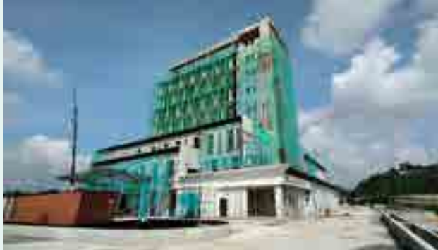
Latest Progress for Sepang Medical Centre.
